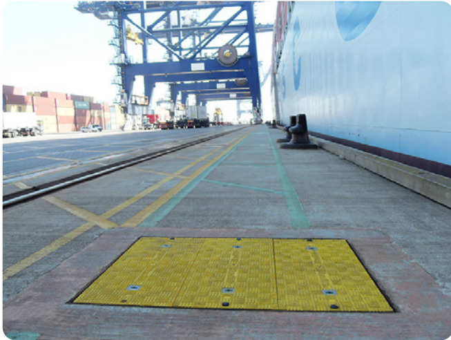
The Fibrelite 90 tonne load rated lightweight trench covers in position on the quayside
