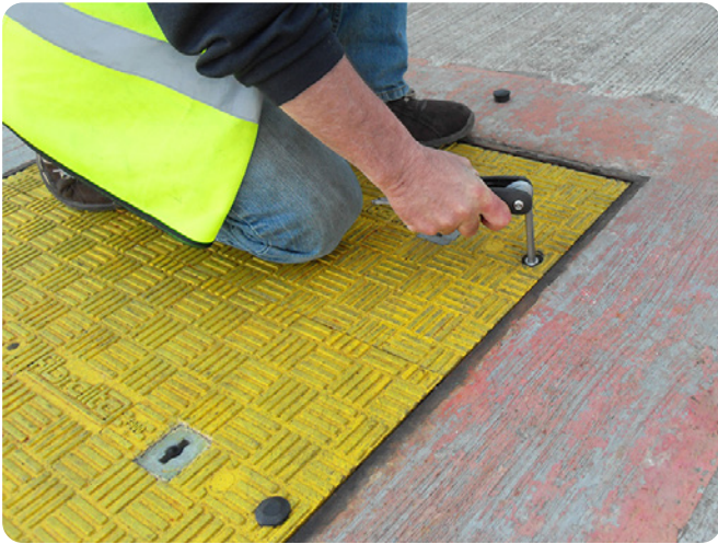
Operator removing the Fibrelite securing system
